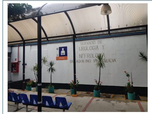
Figure 1. External wall of the Urology Service 105-A.
