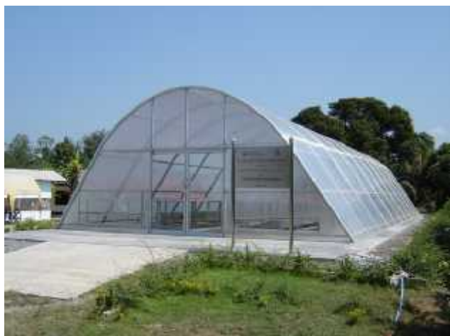
Figure 1. Greenhouse solar dryer designed by Janjai (2012) for small-scale industries.
