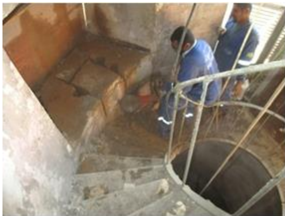
Figure 7. Sample removal process using double diamond disc.
