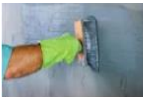
Figure 17b. Primer application as surface preparation
