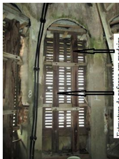
Figure 3. Reinforcement in tower columns
