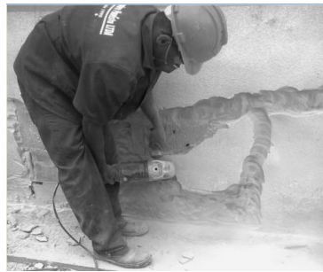
Figure 16a. Roughing process with grinding wheel
