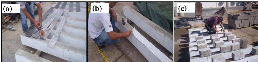
Figure 3. (a) Preparation of the sheets; (b) Application of the epoxy structural adhesive; (c) Fixing and support of the sheets.
