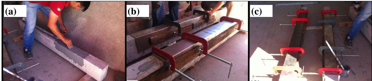
Figure 4. (a) Application of the epoxy adhesive to anchor the steel profiles; (b) Placement of the fasteners; (c) Final fastening system of the sheets.
