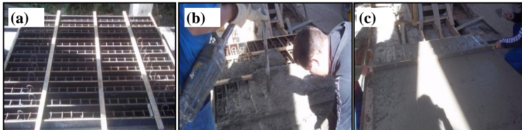
Figure 2. Manufacture of the reinforced concrete beams – (a) Molds with the reinforcement ready for casting; (b) Casting and vibration; (c) Leveling of the concrete in the molds.
