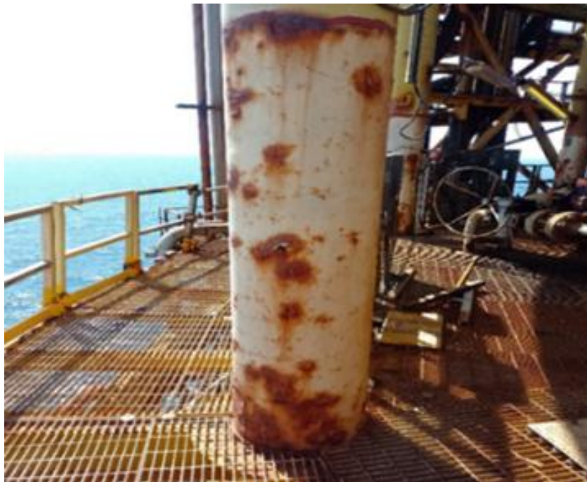
Figure 3. Alveolar corrosion.
