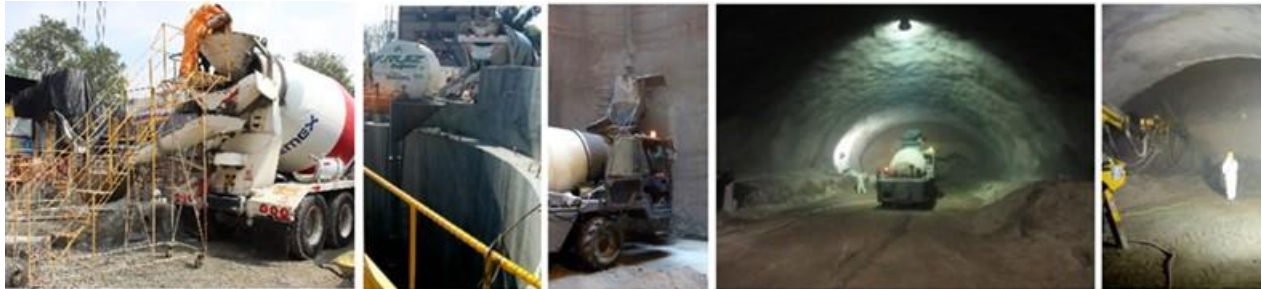
Figure 1. Primary lining placement procedure in L-12 tunnel
