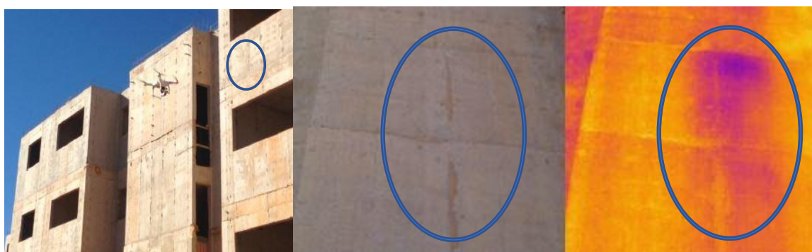
Figure 5. Inspection using an UAV integrated with a thermal camera (Nascimento, 2014)
