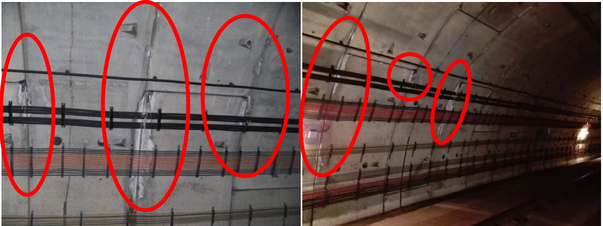
Figure 5. Filtrations (leachings of cement limes).
