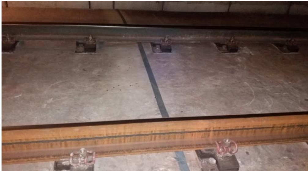
Figure 10. Optical fiber protected under train tracks.
