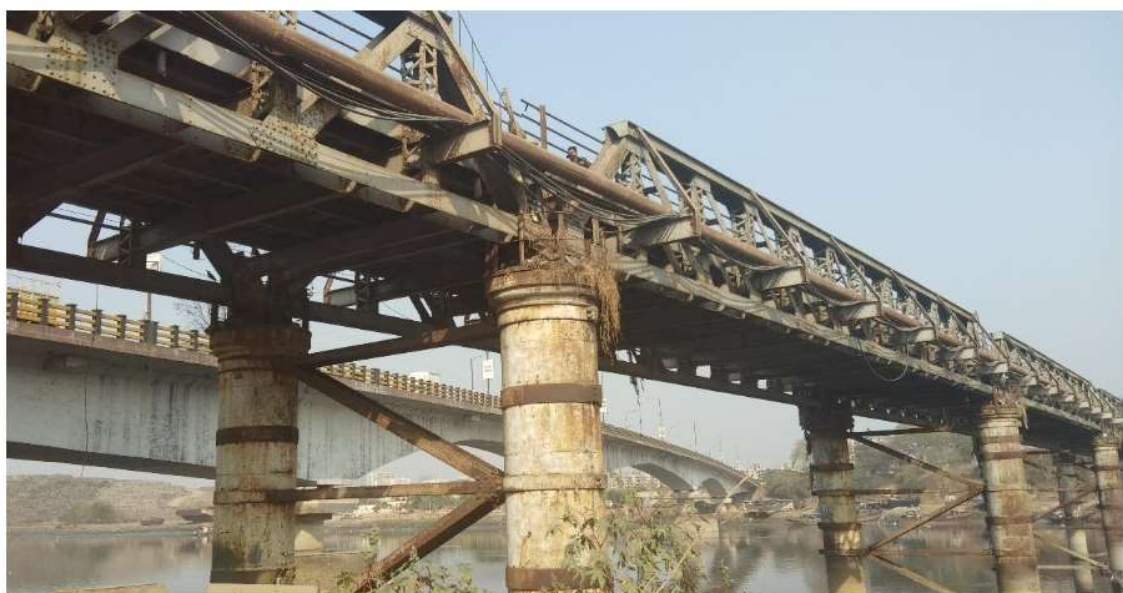
Figure 3. Photo of bridge showing warren truss type structure.
