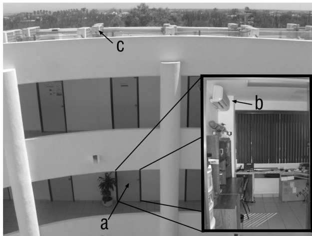
Figure 4. Experimental facility: a) office location, b) minisplit in office interior, and c) minisplit compressor.
