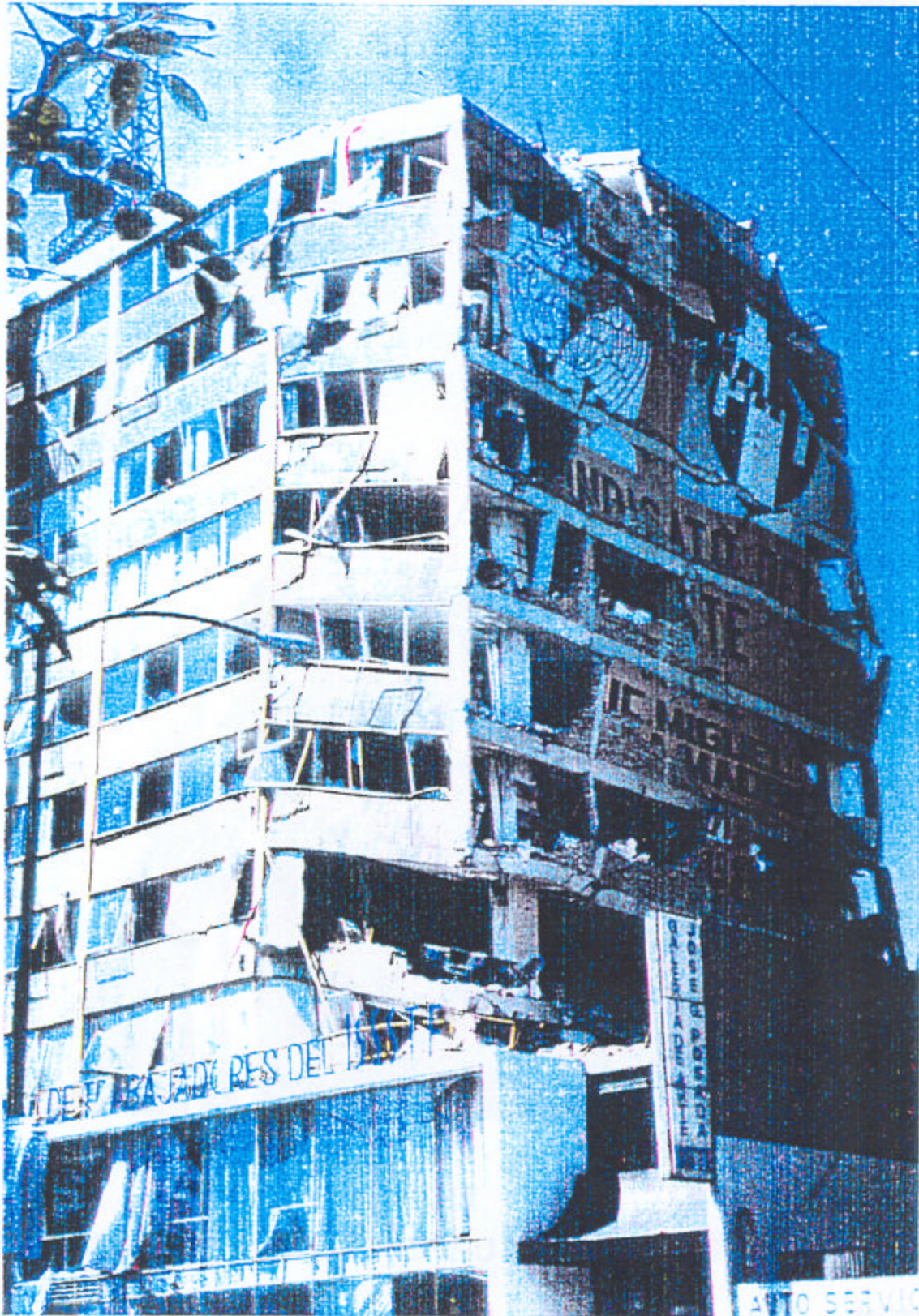
Photo 3. "Whip ping effect" in the upper floors because of seismic action
