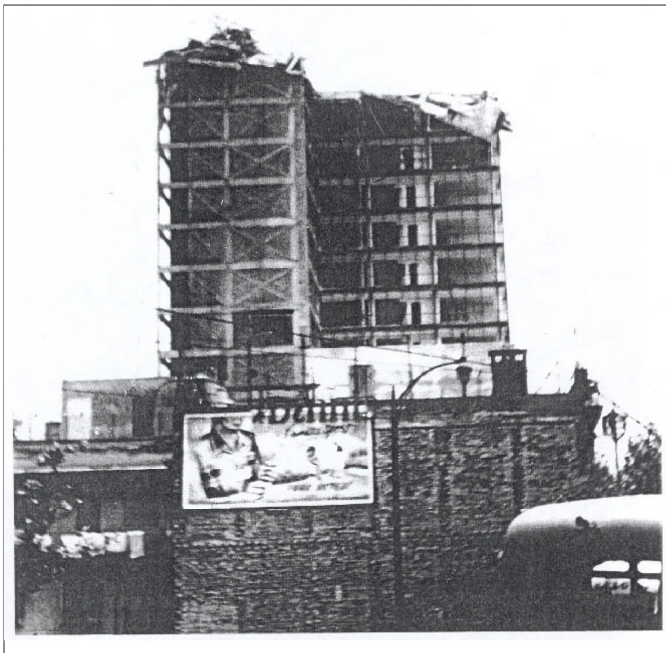
Photo 2. "Whip ping effect" in the upper floors because of seismic action
