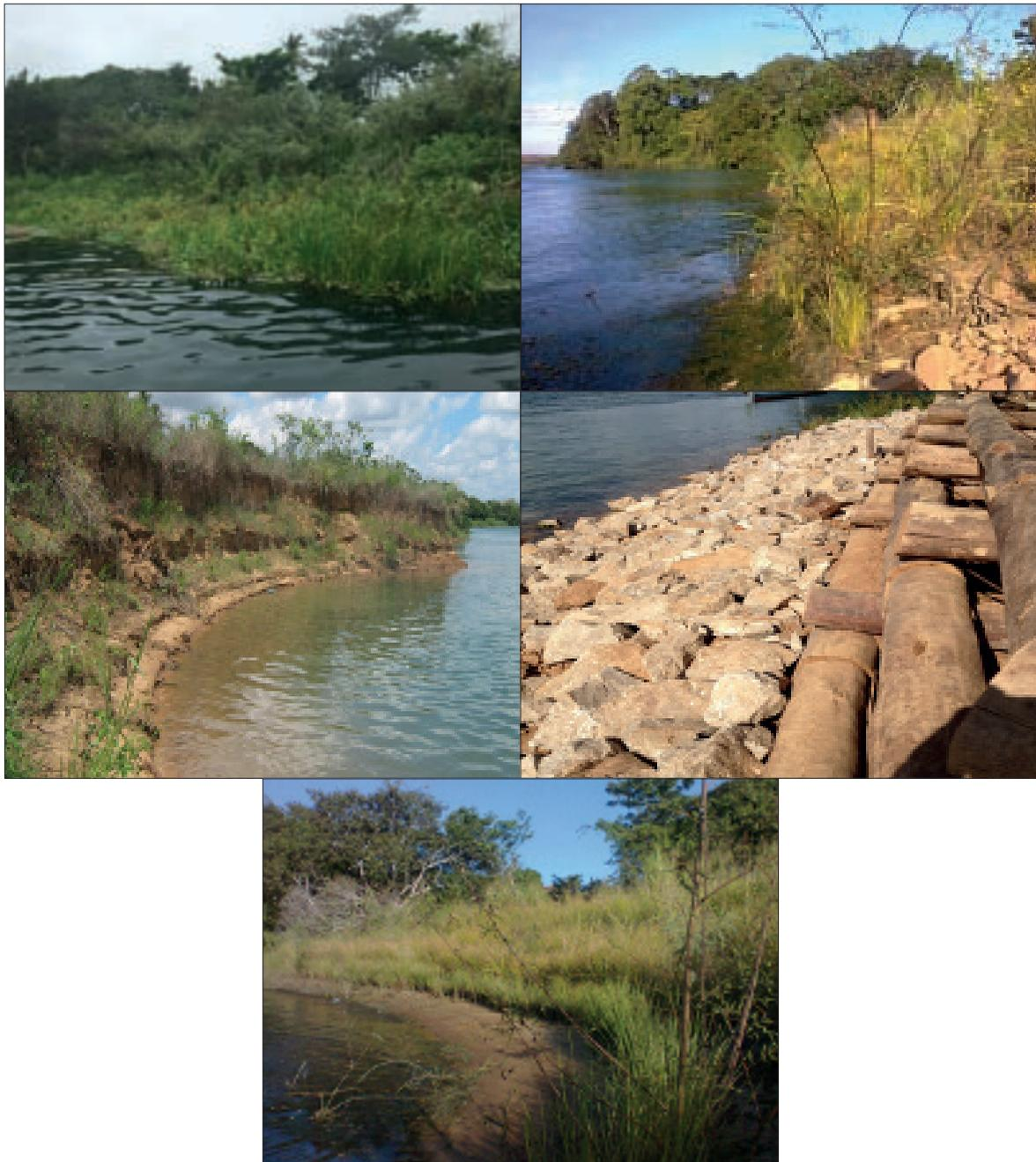
Figure 3. Evaluated treatments: Vegetated slope (a), Vegetated riprap (b), Eroded slope (c), Live cribwall (d) and Vetiver grass contour line (e).
