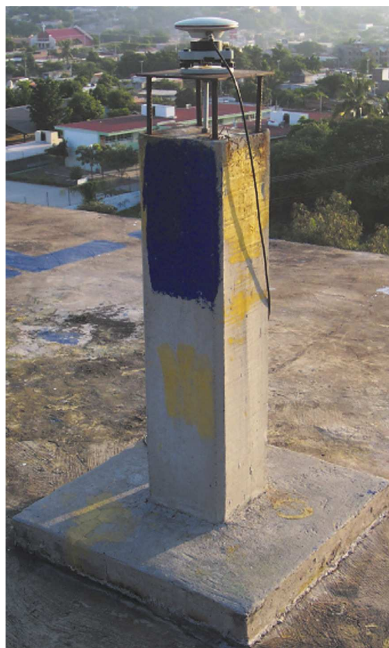
Figure 3. Monumentation of BASE 2 site, located on top of a facility building; UAS campus. GPS Receiver Leica SR500 with Leica (LEIAT502) antenna, collecting data on October 10, 2010.
