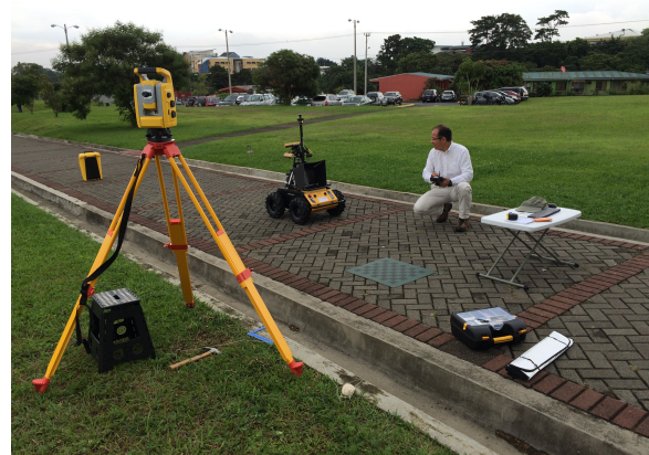
Fig. 1. Clearpath Robotics™ Husky A200™ rover platform and Trimble® S3 robotic total station used for experimental validation
