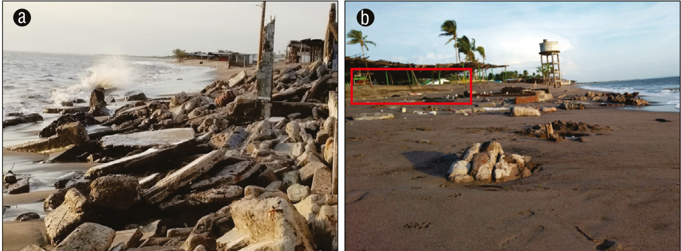
Figure 8. Impact of sea level rise on the coastal infrastructure of Cedeño, Pacific coast of Honduras (PCH). Submerged infrastructure due to sea level rise (a) and coastal erosion labeled in red and local businesses destroyed by sea level rise (b).
