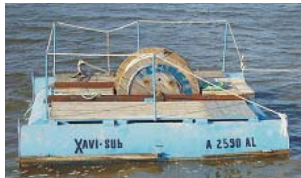
Figure 13. Floating raft used for installing the optical cable.
