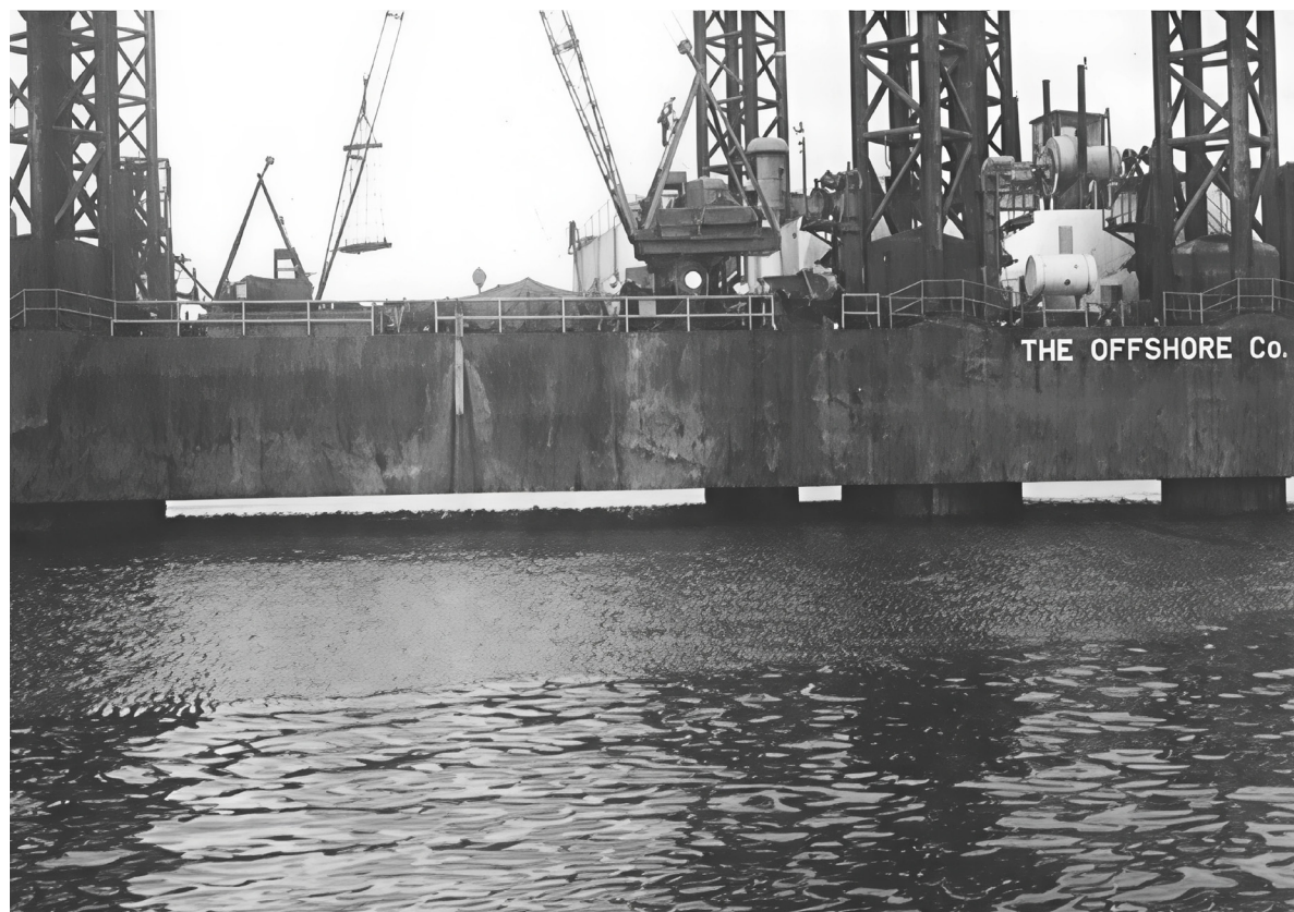
Figure 14 Almirante No. 1 well being drilled in the shallow water of Almirante Bay in 1958 by an early jackup rig, probably Offshore Company Rig 54 or Rig 55, for Champlin Oil (photograph courtesy of Joyce Robinson and Stanley Heckadon-Moreno).
