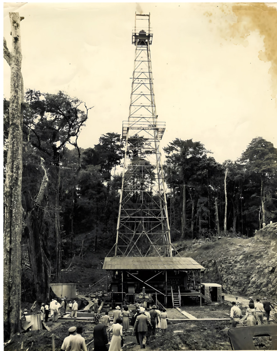
Figure 10 Drilling rig being rigged up to drill Bocas del Toro No. 1 in 1947. The block-line has not been installed yet (photograph by Abraham A. Balid, courtesy of Simon Balid).
