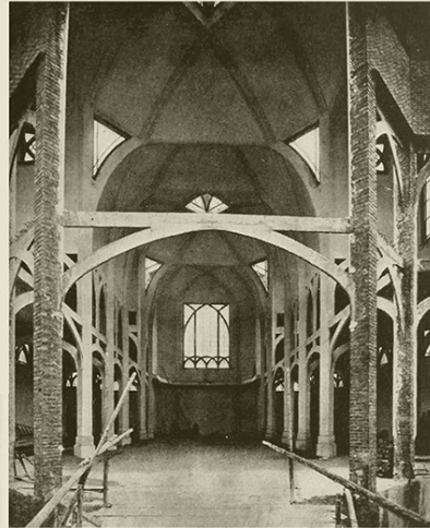
195. ANATOLE DE BAUDOT. Saint-Jean de Montmartre, Paris. Begun 1894. The first church to be built with a ferroconcrete skeleton closed in by thin outer walls.
