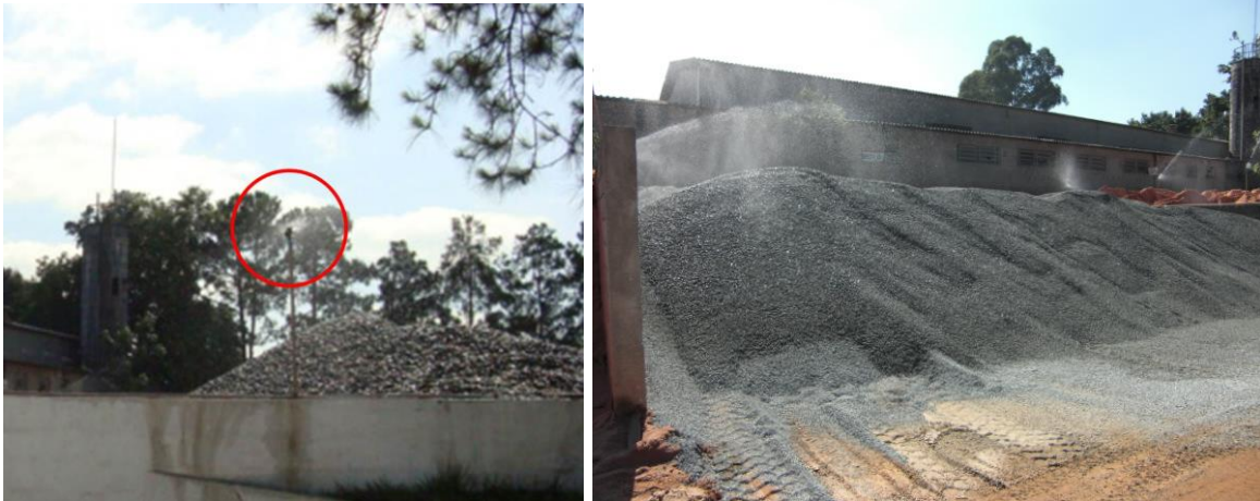
Figure 6. Coarse aggregate being water-sprayed at Ready-mix Company batching plant.
