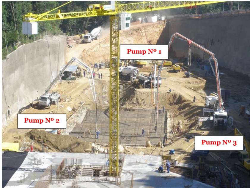
Figure 10. General view – Concrete pumps positioned.
