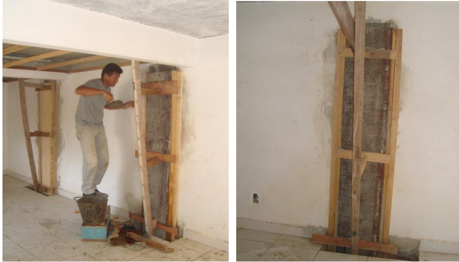
Figure 9. Concrete casting of the structural strengthening.
