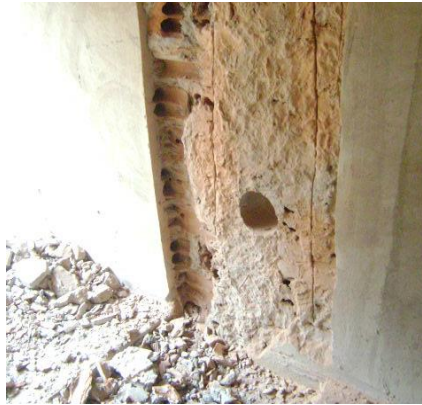
Figure 4. Testimonies' extraction hole in a column.
