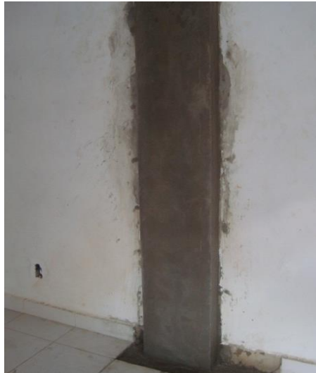
Figure 10. Final aspect of the strengthened columns.
