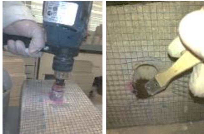
Figure 3. Extraction of cylinders and dust samples.
