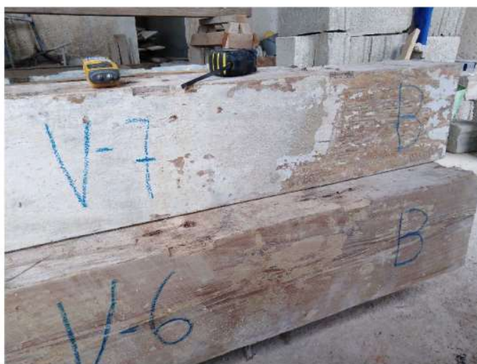
Figure 8. Identification of wooden beams
