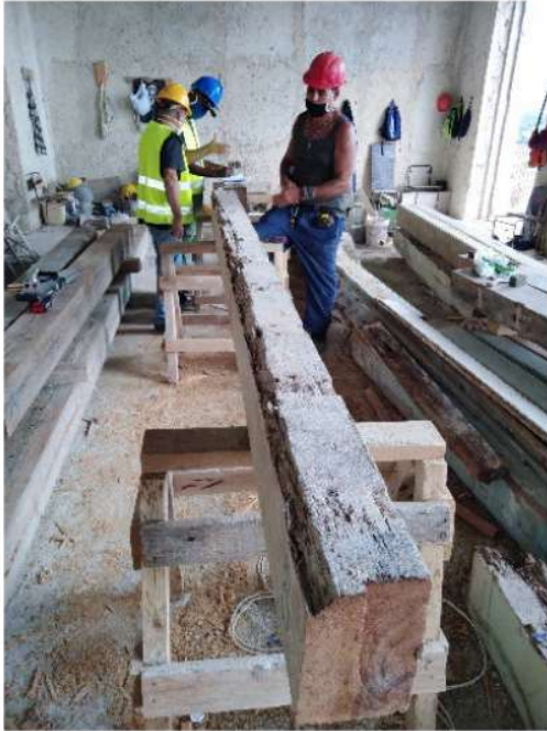
Figure 3. Stage of detailed inspection in beam mounted on wood supports
