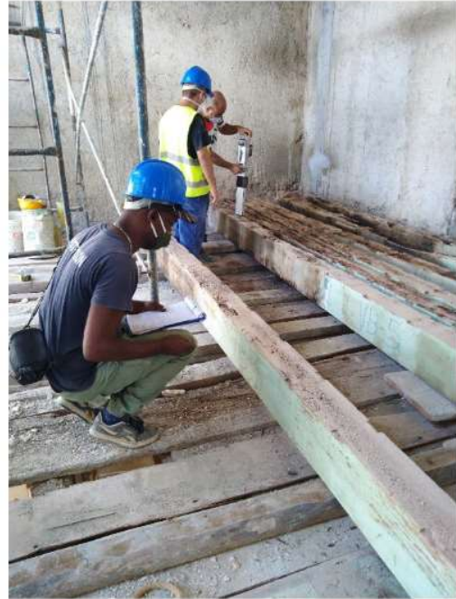
Figure 4. Inspection and visual classification of disassembled beams
