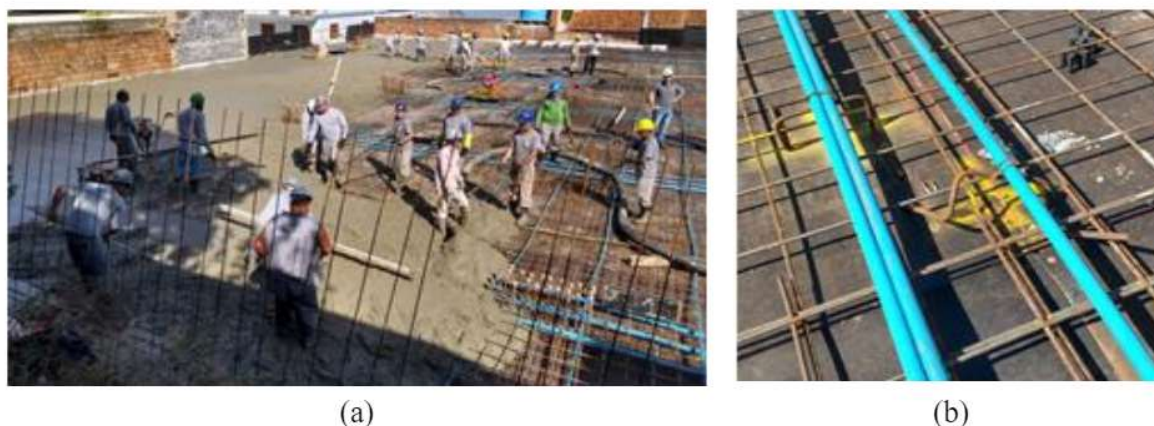
Figure 1. Concrete pouring example: (a) workers in direct contact with the reinforcement and (b) damaged and out of position spacer.
