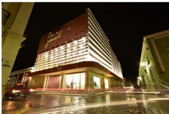
Figure 7. View of the intervention building
