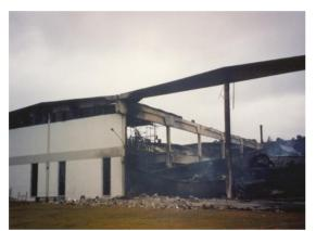
Figure 11. Collapse of building with precast structure subjected to fire
