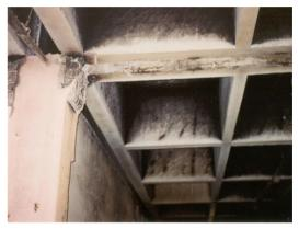
Figure 12. Support displacement of premolded fire structure
