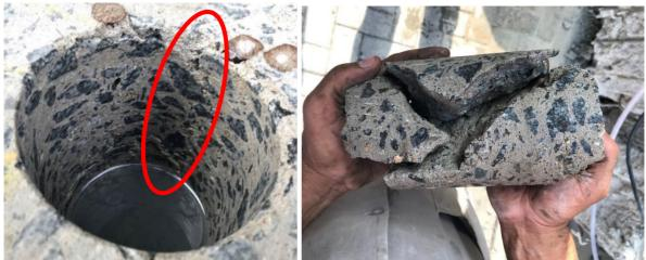
Figure 13. Visible cracks during extraction and decomposed core. (Source: Paulo Helene's personal collection)
