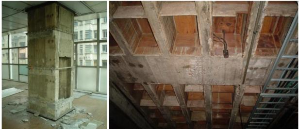
Figure 6. Columns without metal coating, where it is observed the "H" which is actually a shaft of the air conditioner and l grate beam track with AJE still forms wood. (source: personal collection of Leandro Coelho)
