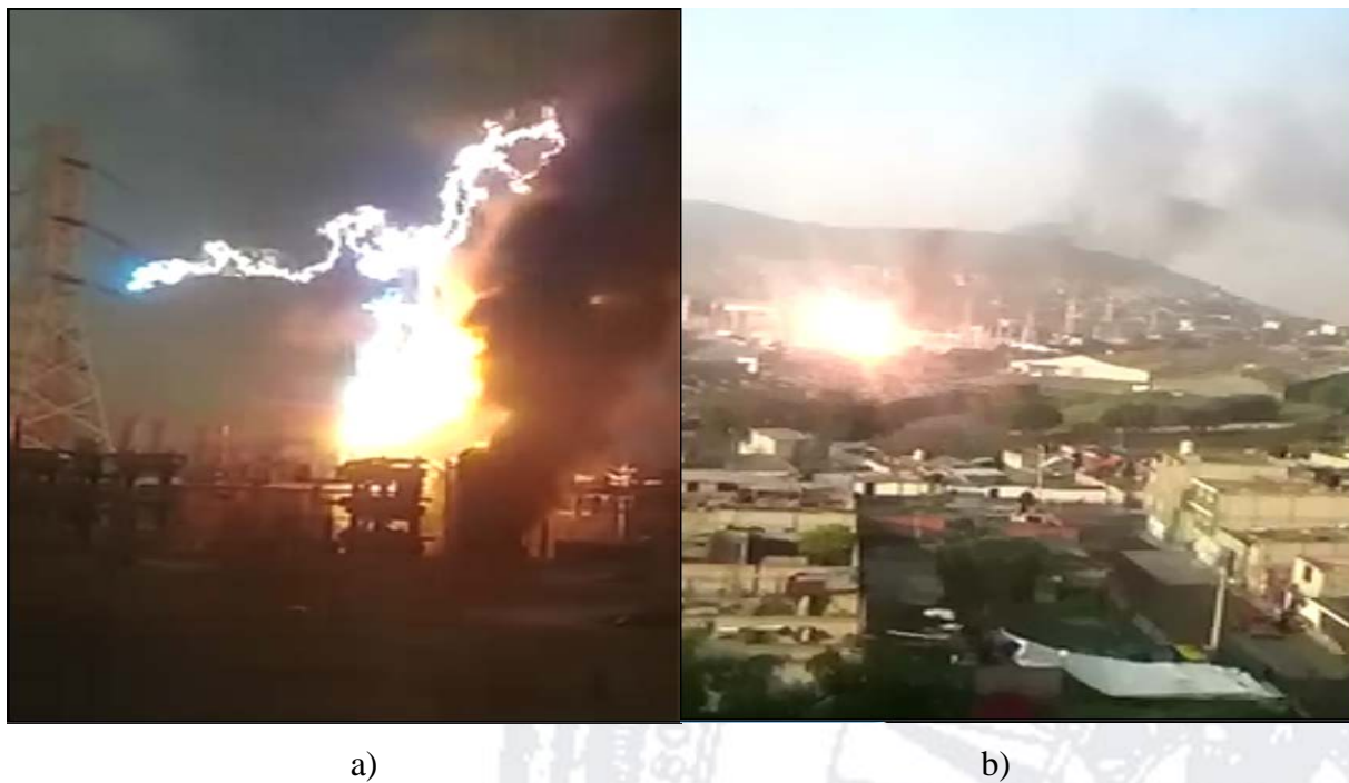
Figure 25. a) Electric arc due to overvoltages in SVC of Cerro Gordo substation, instant of the explosion, picture is taken inside the substation. b) Explosion in Cerro Gordo substation picture taken from a apartment building.
