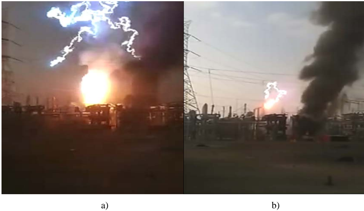
Figure 24. a) Electric arc due to overvoltages in the SVC of Cerro Gordo substation of 230 kV. b) Electric arc due to overvoltages in the SVC of Cerro Gordo substation of 230 kV.
