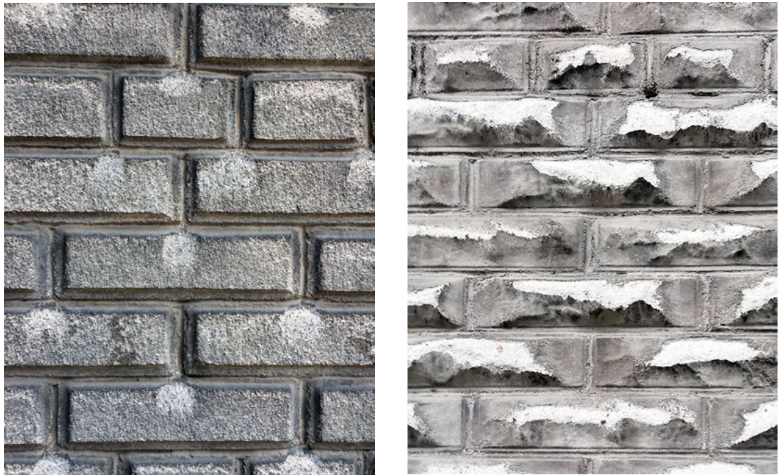
FIGURE 2. Two types of cement bricks (20 x 10 x 6 cm). Left, detail of smooth partition wall rigging with bevel; right, detail of grotesque partition wall rigging with bevel (Photographs: Alejandro Leal & Alberto Muciño, 2020; source: Authors' Collection).
