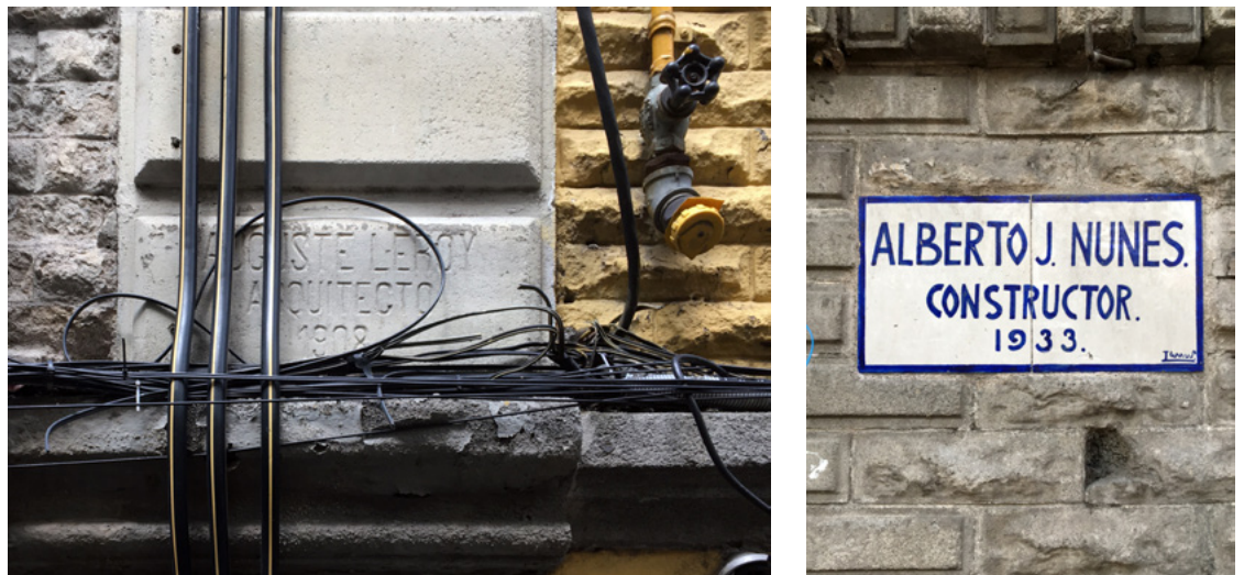
FIGURE 8. The dates of these two photographs comprise the first and last dates found in the field (in 2021) that verify the use of cement partition walls in Mexico City. Left, authorship signature of architect Auguste Leroy dated 1908; right, authorship plaque of builder Alberto J. Nunes dated 1933 (Photographs: Alejandro Leal & Alberto Muciño, 2021; source: Authors' Collection).
