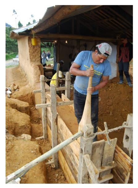
ter, lacks the necessary cohesiveness to preserve its shape, and thus simply cannot be molded. The material, as it continues to be tossed from hand to hand, is continuously kneaded by the process until finally, when it is integrated into the structure, the builders walk over the partially hardened layers and hit them to give uniformity to the lateral faces, as well as to verify and correct their verticality and the leveling of their line (Weismann & Bryce, 2010, p. 150).
