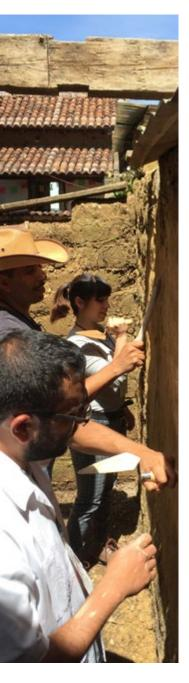
FIGURE 12. Practice of consolidation and re-burial using modeled soil in the classes of the Master's Degree in Conservation and Restoration of Built Heritage of the ENCRYM-INAH (Photograph: Luis Fernando Guerrero Baca, 2019)
