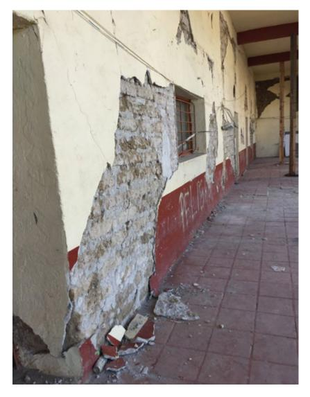
An additional disadvantage, which had not manifested itself so dramatically, derives from the fact that, when seismic movements occur, concrete surfaces crack very easily due to their rigidity, while the adobe structures remain stable inside, as they have greater
