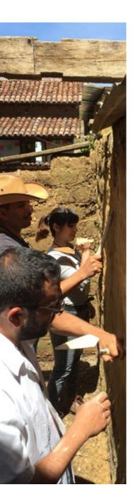
sequent compaction was demonstrated. These procedures make it possible to carry out coatings and build thin walls for conventional works.
