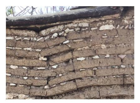
Data on the compressive strength of adobe fractions that have been analyzed in the Laboratorio de Materiales of UAM-X and the indication of load bearing capacities from 4 to 7 kg/cm2 may give the idea of an apparent weakness. However, in reality those pieces have formed the walls of historical buildings in Calpan, Puebla; IXtepec, Oaxaca; Hueyapan, Morelos, and Cocóspera, Sonora, and resisted gravitational pressures and accidental stresses for centuries.
