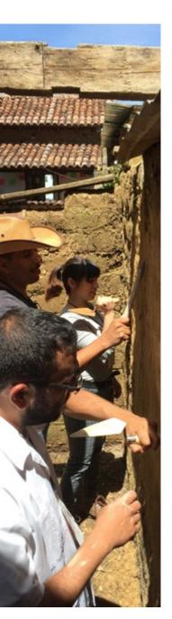
is again moistened with a sprinkler and the next series of spheres, which constitute the second layer, are applied and the operation is repeated. In this way, the holes are covered with successive layers, but with a gradual progression that guarantees their adequate adherence and the successful sealing of possible internal cavities, recovering the unity of the restored component (Figure 10).
