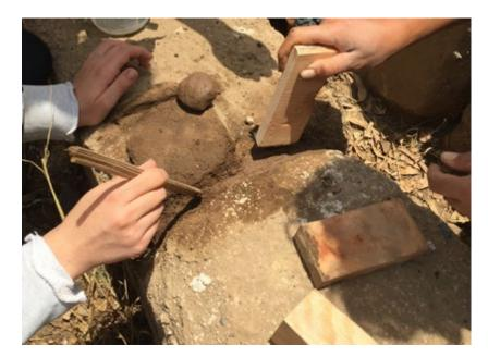
If the damage to the walls is very deep, such as in continuous fissures or cracks, equidistant tubular "nozzles" can be inserted over the entire length during the filling and compacting process. Once the closing of the crack is completed, a fluid clay paste stabilized with 5 to 10% in volume of calcium hydroxide is injected, which will be gravitationally distributed within the cores. Finally, the nozzles are extracted or cut away and the operation is completely sealed.
