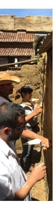
ductility. In addition, since they are joined with mortars that are also made with mud, they absorb significant deformations without cracking (Guerrero & Vargas, 2015, p. 64).
