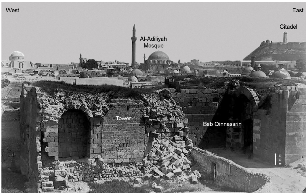
Figure 7. A photo of Aleppo dated back to 1890 showing Bab Qinnassrin, one of two southern gates of the city. Note the remains of its tower destroyed by the 1822 earthquake. Source: Historical Digital Documentation House in Aleppo at: https://www.dig-doc.org/images/photo_gallery/pic_36202052727.jpg
