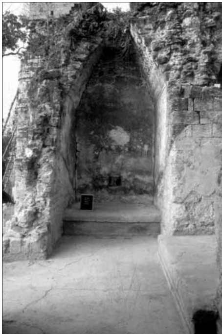
FIGURE 12. Bench and wall niche, south end of Room C
