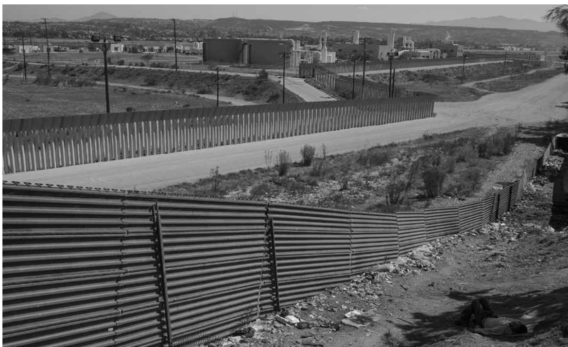
PROMETEO LUCERO ▶ Muro fronterizo, Tijuana.
