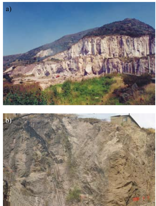
Figure 7. Anthropic modification of relief. a) Quarry zone, showing vertical walls and vehicles working near of the zone. b) House built adjacent to a steep wall (old quarry).
